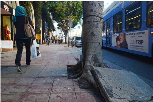
Figure 3.5 Roots lifting slab of concrete. (Photograph courtesy L. Atmore, Daily Bruin, UC Davis)
